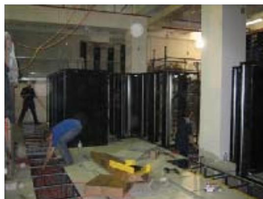
Image: Data Centre under construction. Raised floor provides good access
